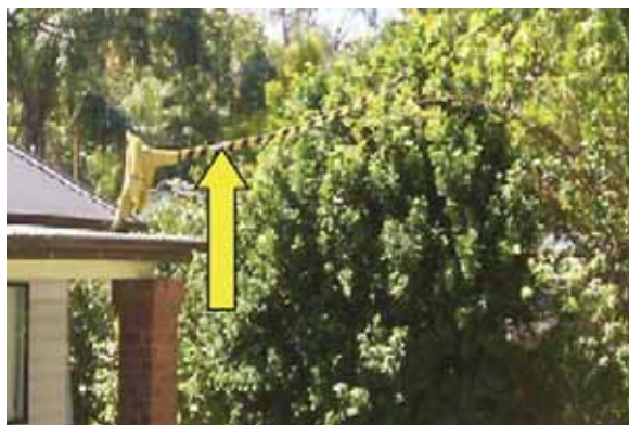
Figure 15 – Insulated matting and tiger tail fitted to overhead service line
