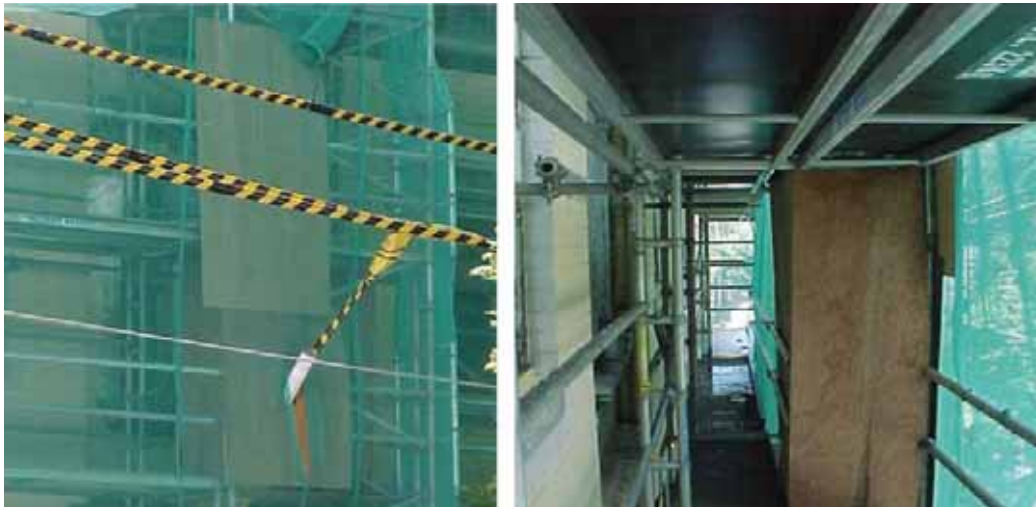
Figure 11 – Enclosure of overhead powerlines
