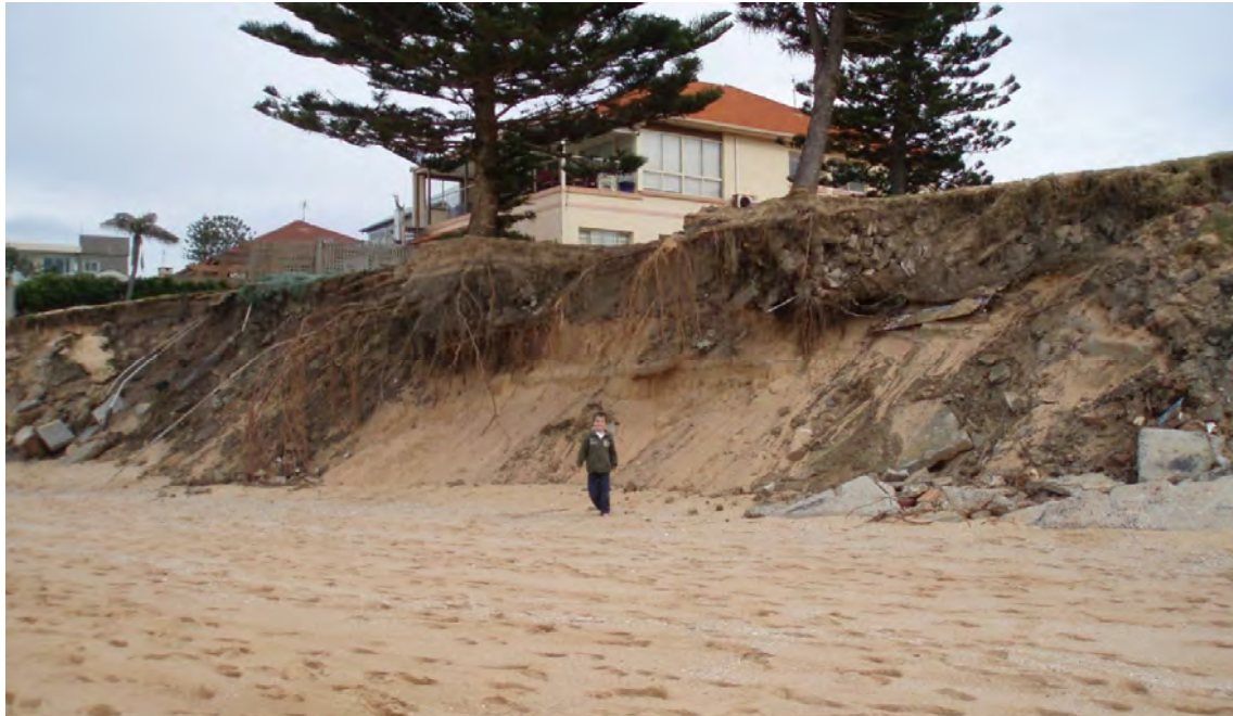
Figure 6: Undermining of pine trees at 1184-1186 Pittwater Road Narrabeen, 29 July 2007
