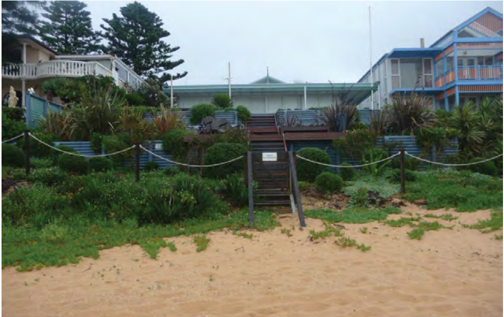
Figure 13: Timber retaining wall at 21 Pacific Street, 22 November 2011
