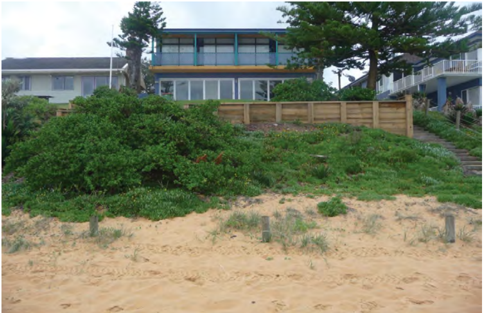
Figure 15: Timber retaining wall at 31 Ocean View Drive, , 24 November 2011
