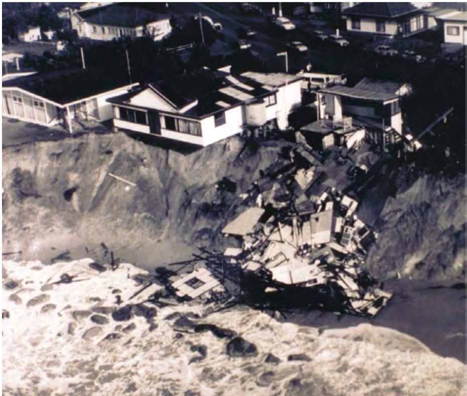
Figure 11: House collapse at Wamberal-Terrigal Beach in June 1978
