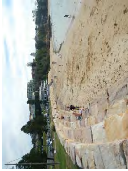
Figure 1: Stepped sandstone block seawall along the southern section of Terrigal Beach (left) and block seawall and promenade along the central section of Terrigal Beach (right)
