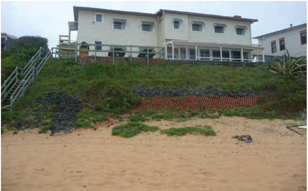
Figure 19: Rock basket and “seabee” protective works at 59-61 Ocean View Drive, 24 November 2011
