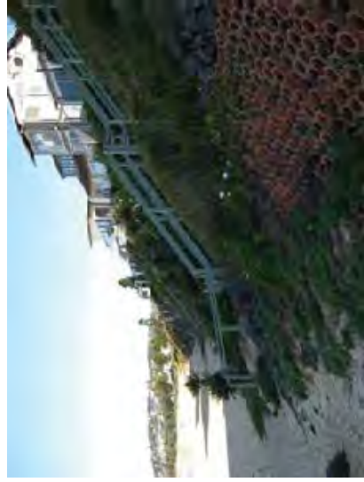
Figure 2: Rock gabion and terracotta pipes (left) and concrete retaining walls (right) constructed in front of properties
