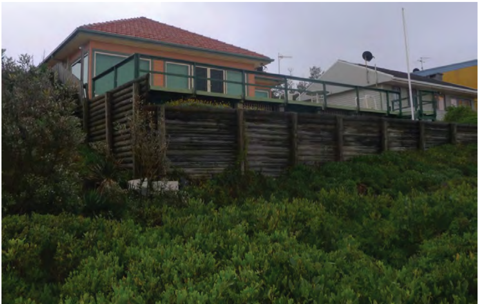
Figure 14: Timber retaining wall at 27 Ocean View Drive, 22 November 2011
