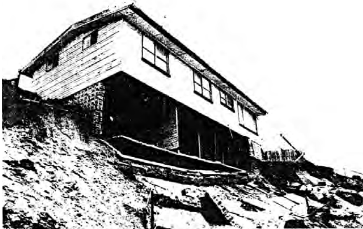
Figure 10: House severely damaged by dune erosion at Wamberal-Terrigal Beach in 1974 (from PWD, 1985)
