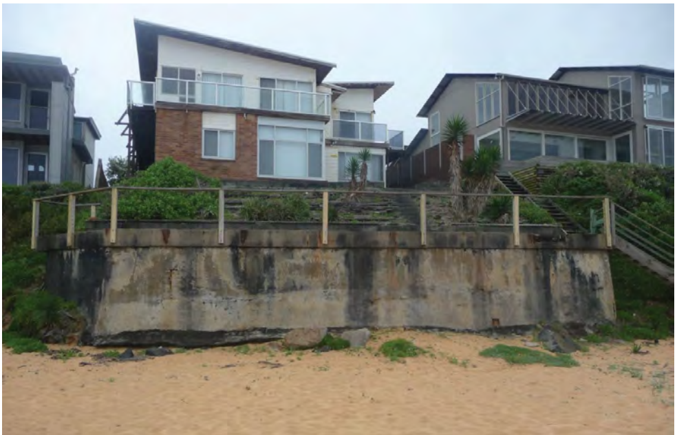
Figure 18: Vertical concrete seawall at 53 Ocean View Drive, 24 November 2011
