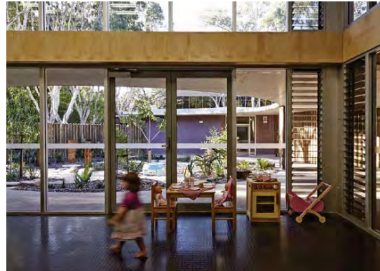
Louvres can be incorporated to allow for ventilation when doors are closed.
