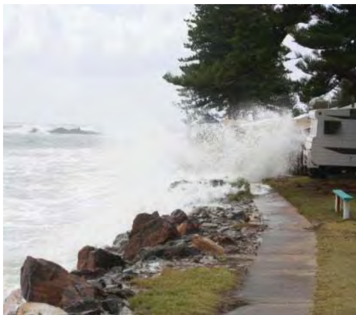
Plate 2 Wave overtopping at southern end of caravan park 25/12/2011 (Mr Mark Cameron)
