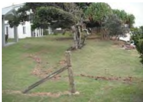
Plate 3 Debris line from overtopping of ad hoc Ocean Rd revetment 6/6/2012 (CVC)
