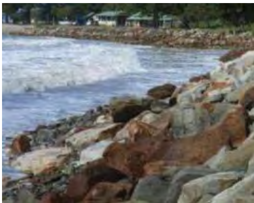
Plate 1 Foreshore Reserve Revetment (22/8/2011)
