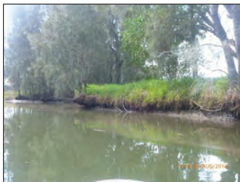
Figure 11(b) Mid estuary bank erosion
