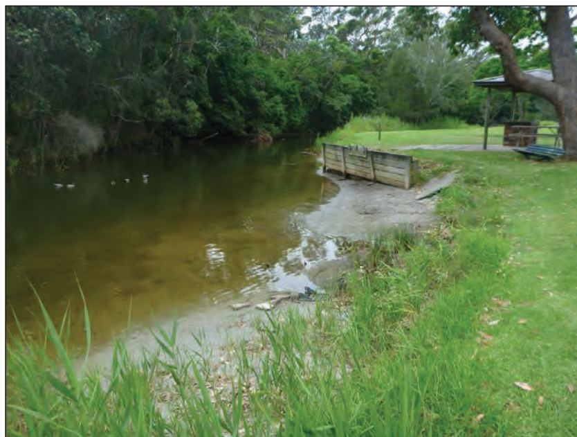
Figure 11(d): Erosion occurring in Blue Angle Creek
