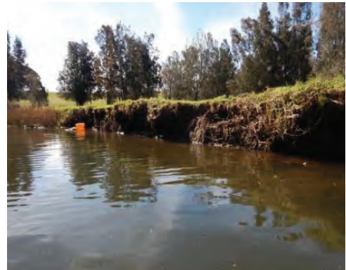
Site 14 – Downstream Swamp Road (D. Wiecek, 2014)
