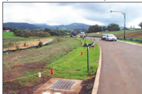
Union Creek riparian works in Elambra Estate
