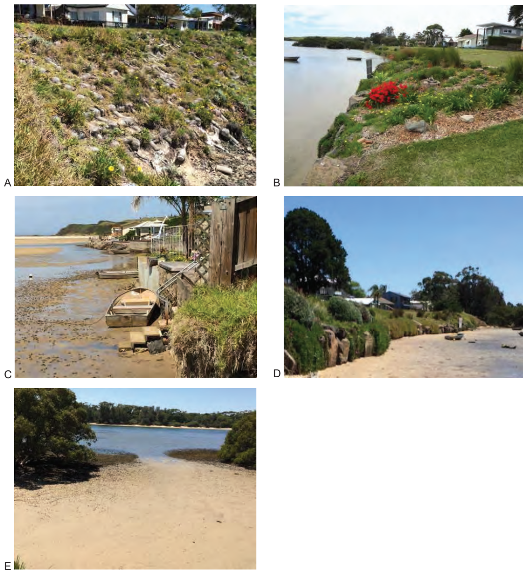
Figure 30: Charles Avenue erosion and existing controls
