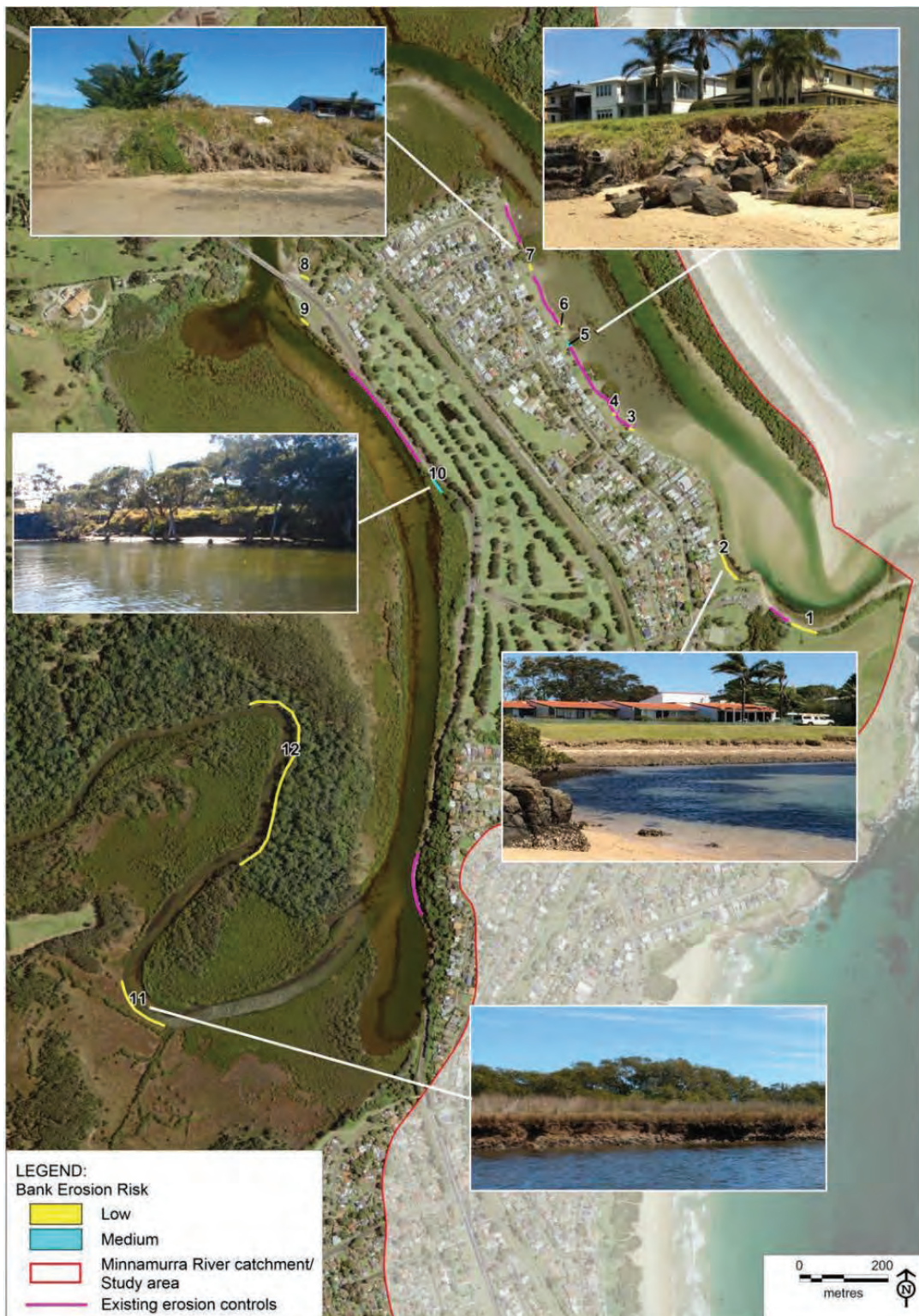
Figure 33: Locations of bank erosion sites in the lower to mid-estuary
