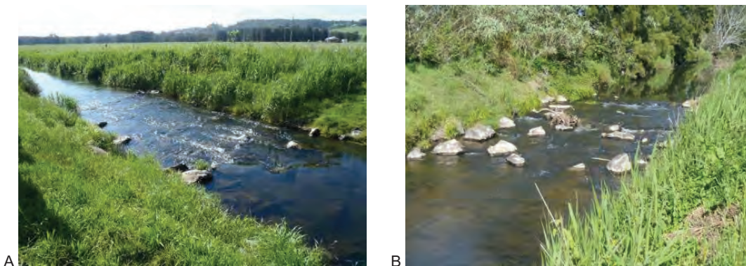
Figure 32: Terragong Drain rock ramps
