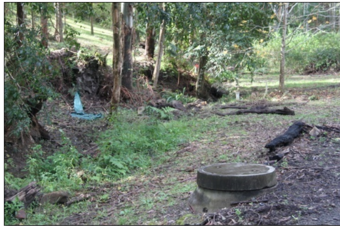
Figure 6-1 Sewer manhole near creek entering Smiths Lake
