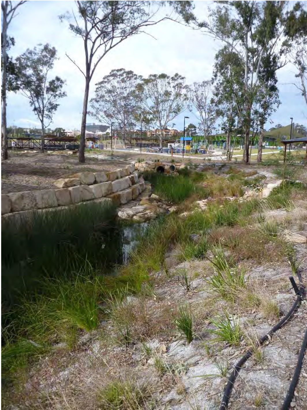
Figure B3.19 An example of water sensitive urban design: vegetated swale with floodway, Bankstown (Photo: P Vella/OEH)
