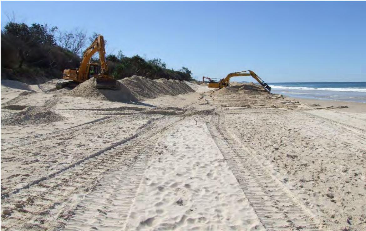
Figure B3.12 Beach scraping at New Brighton Beach, Byron Shire Council (Photo: B Fitzgibbon/Byron Shire Council)
