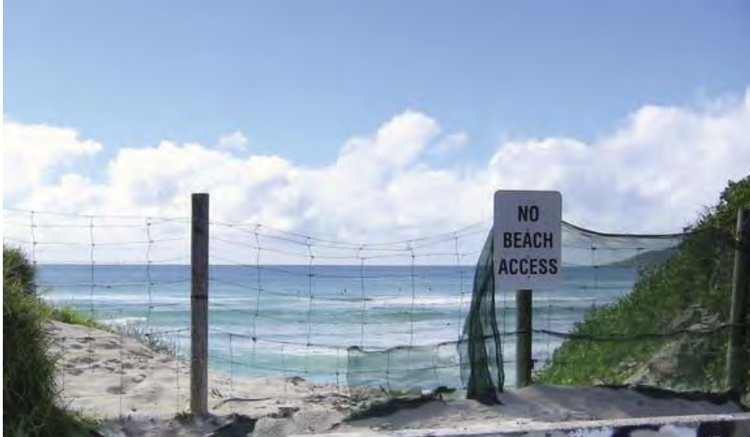
Figure B3.15 Signage and fencing to prevent public access to eroded beach area, Byron Bay (Photo: S Holtznagel/OEH)
