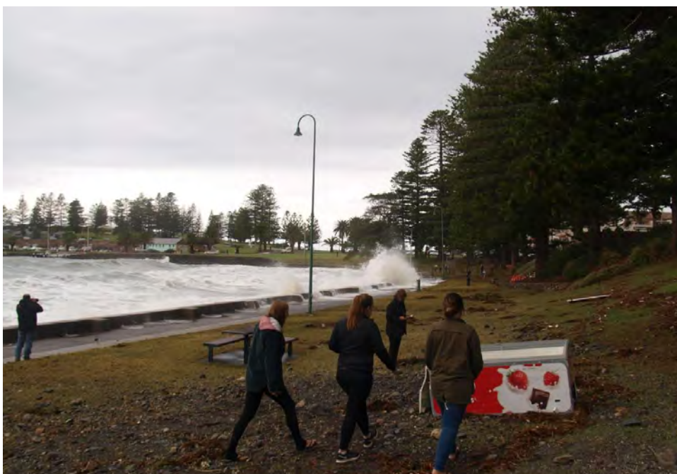
Figure B2.15 Waves overtopping seawall at Kiama Harbour depositing debris on foreshore, June 2016 (Photo: D Wiecek/OEH)
