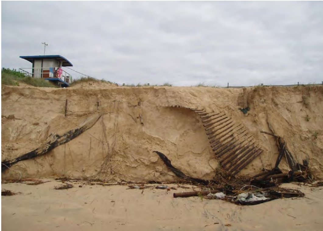
Figure B2.23 Risks to public safety from coastal erosion, Park Beach, Coffs Harbour (Photo: OEH)
