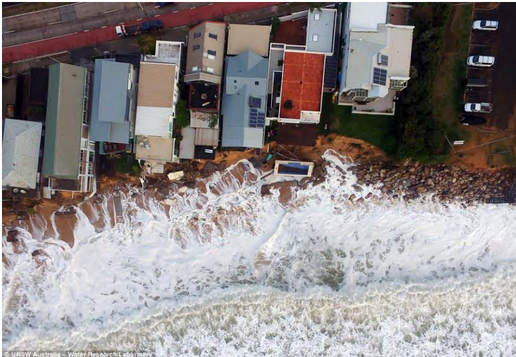
Figure A4 Erosion at Collaroy Beach, June 2016 (Photo: UNSW Water Resources Laboratory)
