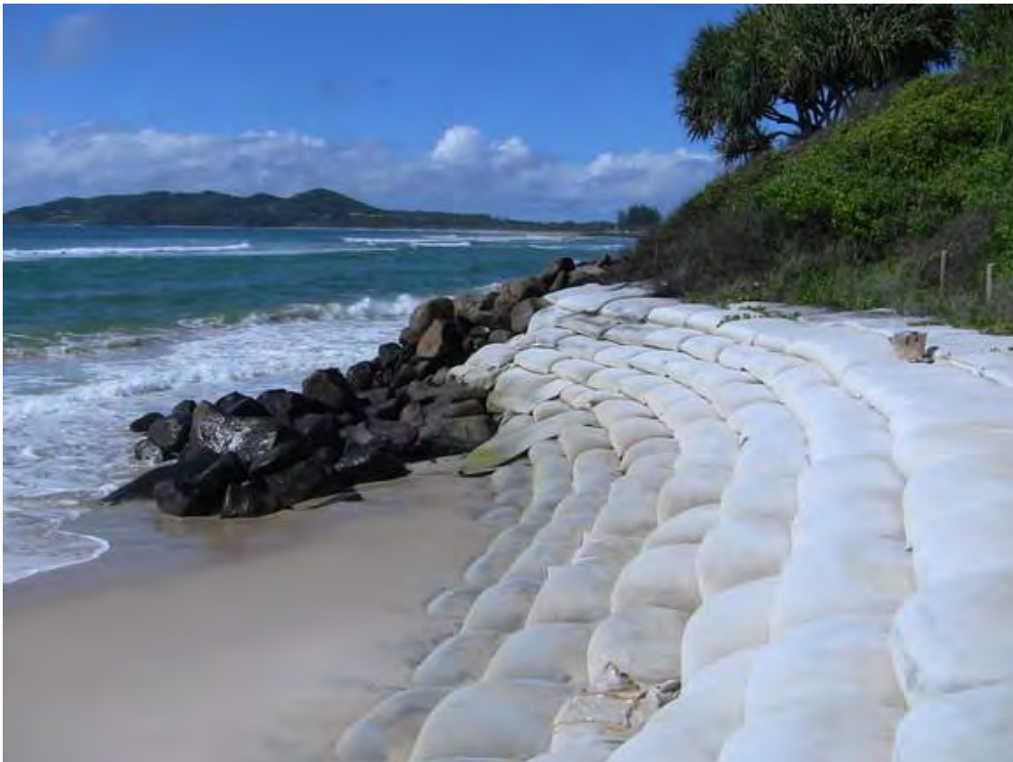
Figure B3.9 Coastal protection works, Belongil Beach (Photo: P Davies/OEH)
