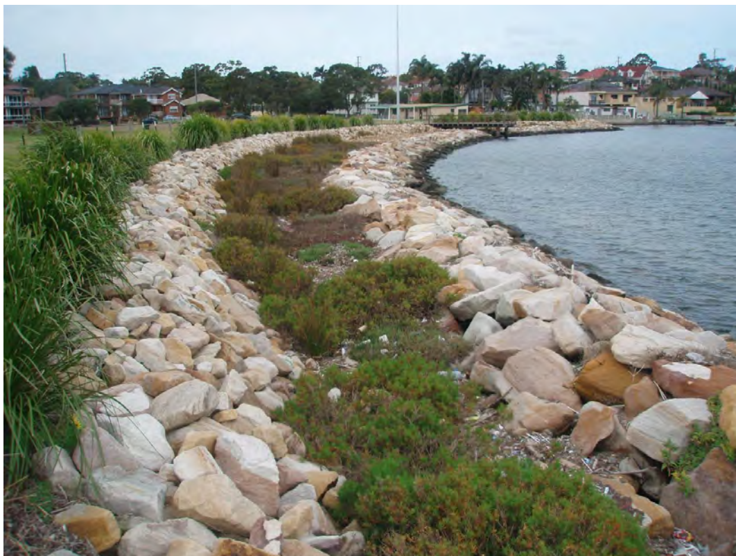
Figure B3.14 Seawall at Kogarah Bay showing step-type seawall with a bench of saltmarsh vegetation (Photo: D Wiecek/OEH)
