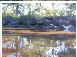
Lower Boambee Creek: right bank showing bedrock base
