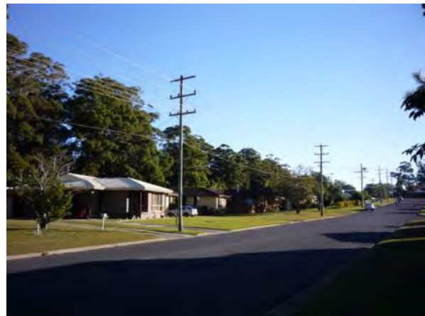
Plate D4.2 Large trees within the tributary reserves offer a highly significant visual resource for the surrounding residential communities
