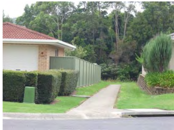
Plate D2.3 Path to nowhere. This pedestrian corridor leads into a hidden area of drainage reserve that offers minimal recreational value and poor passive surveillance
