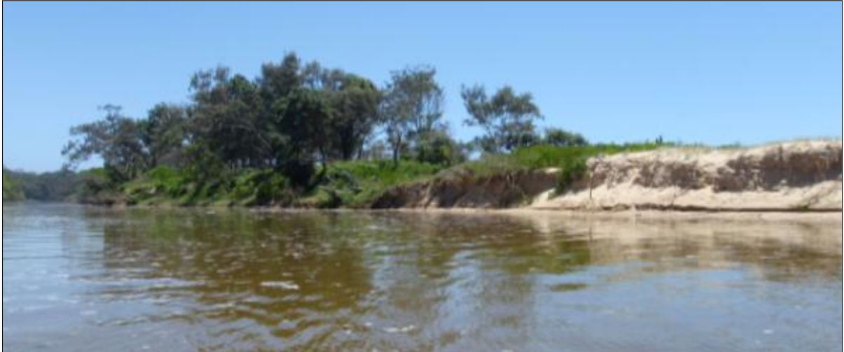
Plate C.3 Bank Erosion - scour and undercutting, lower Darkum Creek – left bank (looking north)
