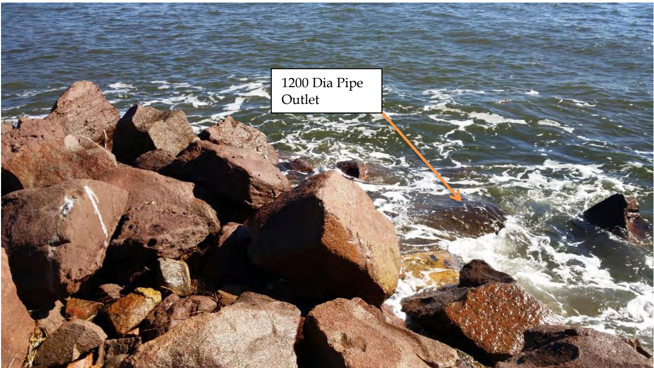
Photo 2 - Outfall 2 Looking north
