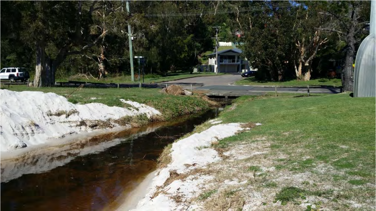
Photo 1 - Looking south towards surcharge pit at Outfall 1 location.
