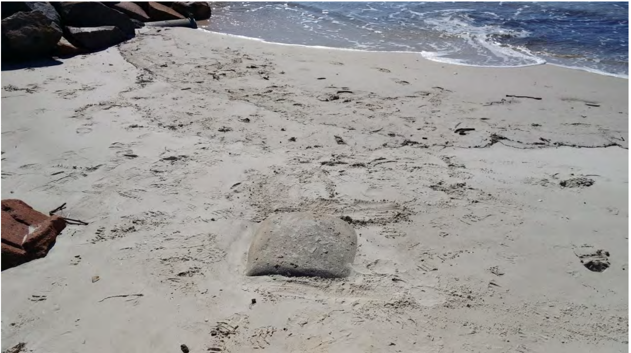
Photo 4 - Outfall 4, completely blocked.
