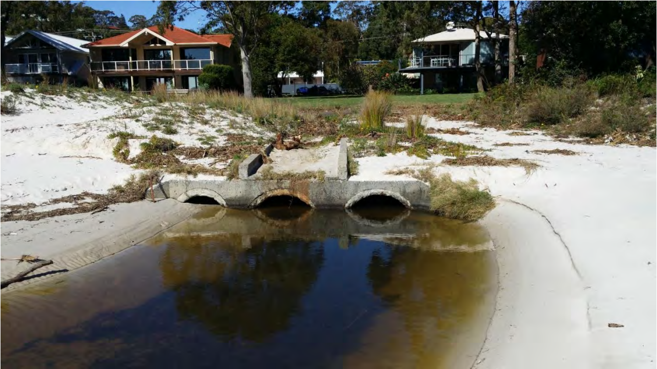
Photo 3 - Outfall 3 Looking South East
