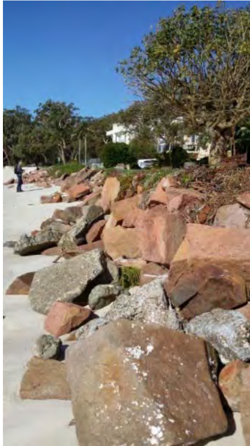
Figure 16 Precinct 6. Some larger rock has been placed along sections of this precinct and a sandy beach remains seaward of this protection work. Photo Source: D Wainwright, 12 th May 2015
