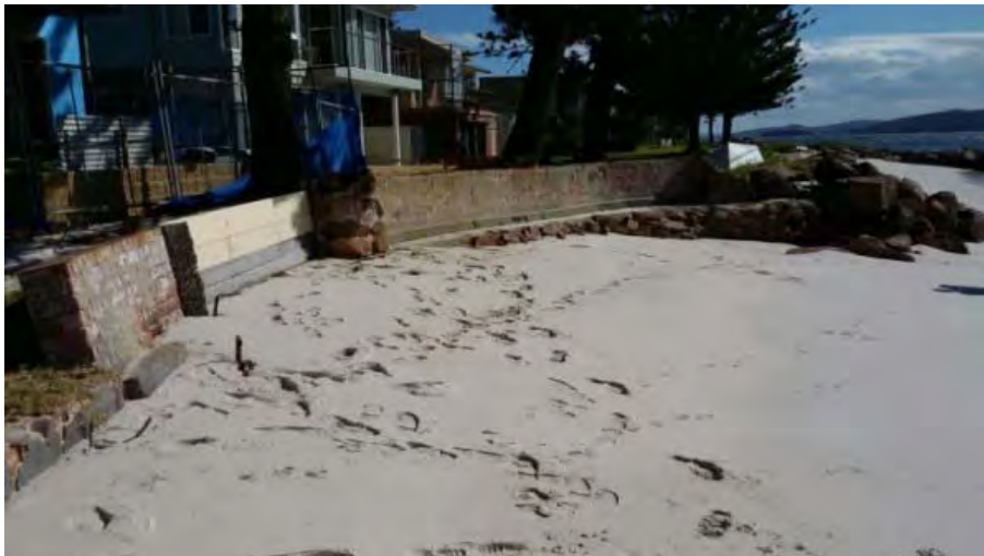
Figure 15 Precinct 6. Located to the east of the eastern most groyne, this section just west of Bagnalls Beach is more sheltered than areas westward (Precinct 5) with generally lower protection structures and a build-up of sand on the eastern side of the groyne. The groyne was lengthened and upgraded to carry the stormwater outlet beyond the beach. The type and standard of back beach protection is variable. Overtopping is experienced right along this precinct although much of the development is set further back from the shoreline. Photo Source: D Wainwright, 12 th May 2015
