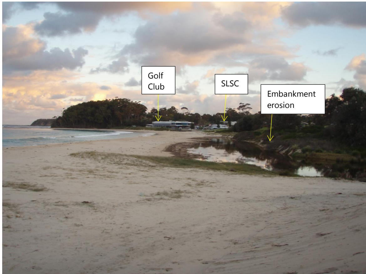
Figure 7 – Southerly breakout of Blackwater Creek causing erosion of embankment and increasing vulnerability of surf club
