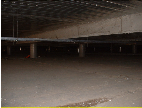
Figure 9 Large vented sub-slab void
