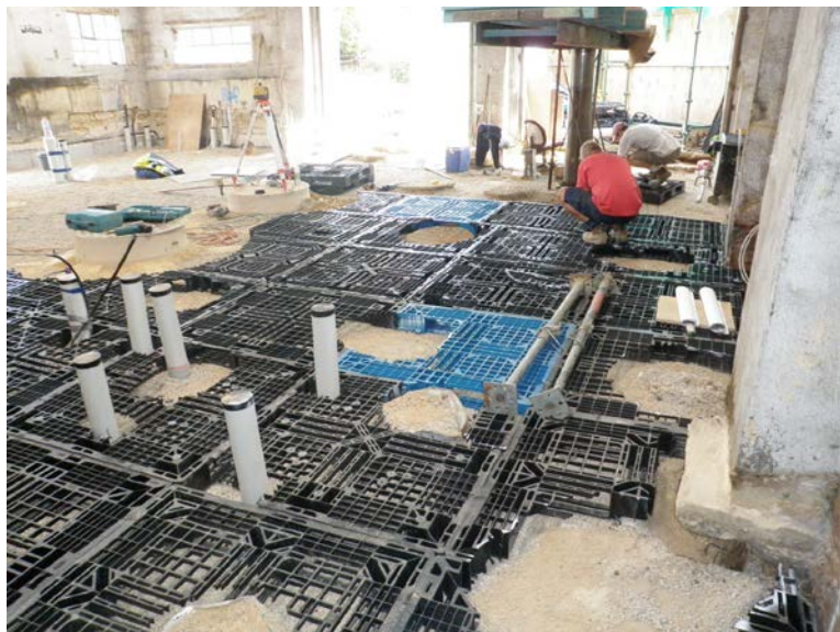
Figure 7 Polypropylene formers create a sub-slab void
