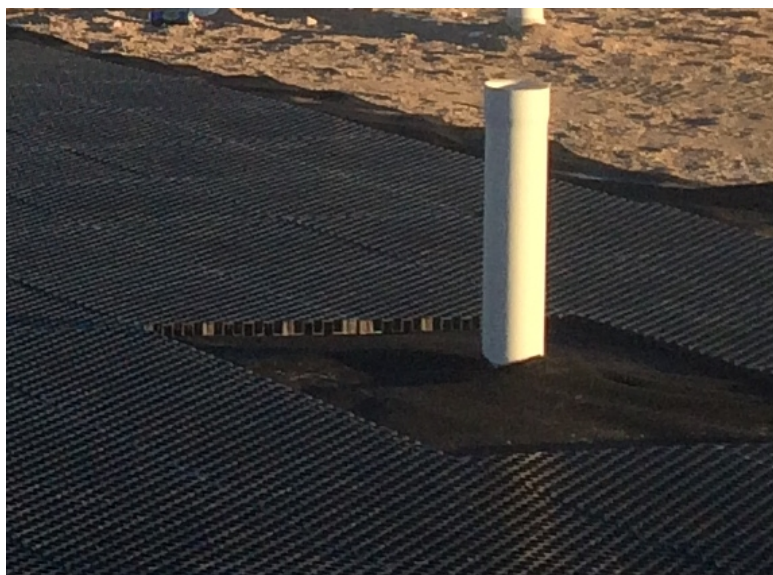
Figure 8 Modular drainage system installed beneath membrane
